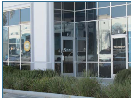
The industrial base in Murrieta is positioned to grow with a range of R&D and light industrial businesses.
